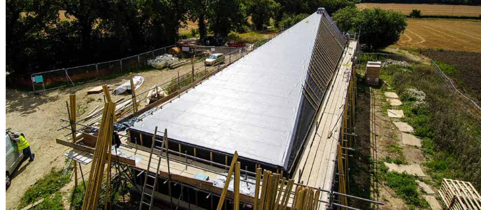
DANOPOL® WATERPROOFING COMPLETED
